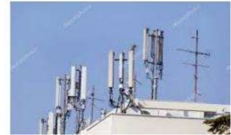
Base stations and antennae on roof top
