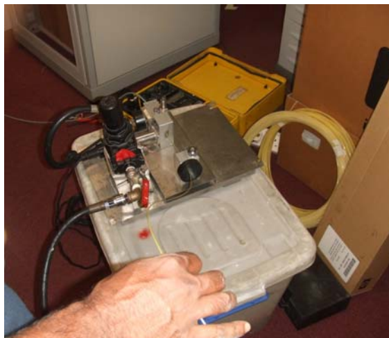
Figure 18: Inserting Fibres into a Microduct (Courtesy of OpenNet Pte Ltd)
