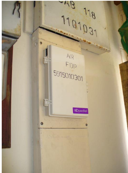
Figure 22: Photograph of a Wall-mounted Fibre Termination Box (Courtesy of OpenNet Pte Ltd)
