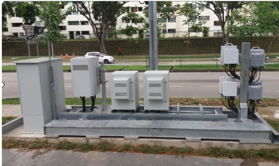
Diagram 2: Example of an Equipment area including the working space required
