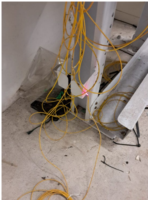
Diagram 4: Example of rodent bites along Singtel's fibre at MDF AM316
