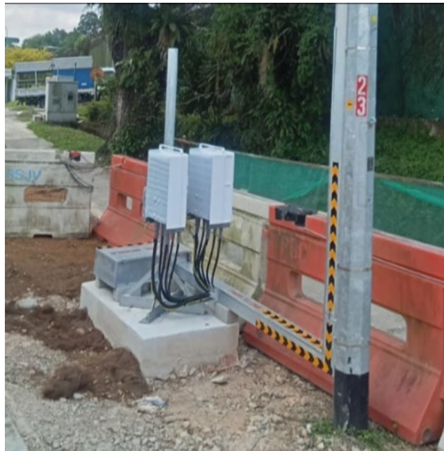
Diagram 1: Example of a Remote Radio Unit
